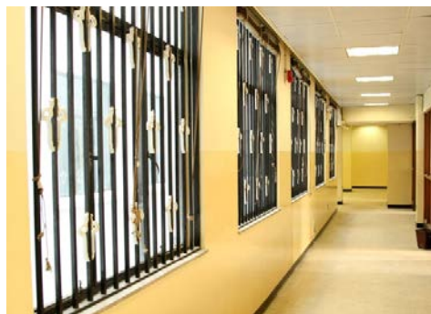
Figure 80 Additional iron grilles at 4/F.
