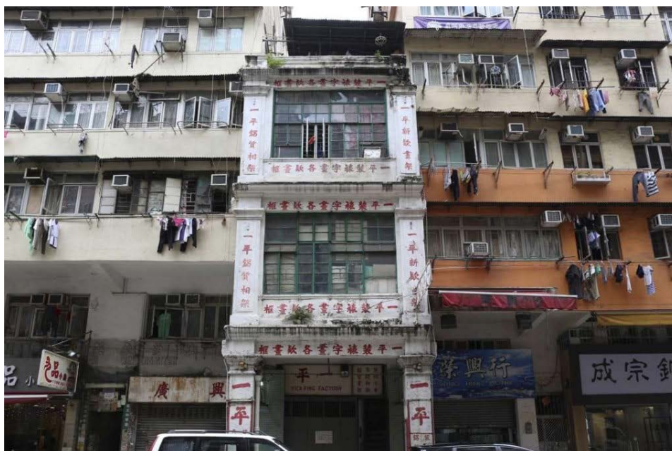
Figure 8 170 Yee Kuk Street, which was built in the 1920s. 29
