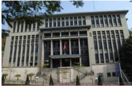
Figure 34 North Kowloon Magistracy before permanent closure. 170
